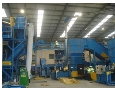
Materials Recovery Facility (MRF) at Longley Lane in South Manchester
