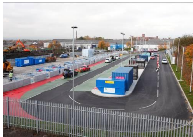
Household Waste Recycling Centre (HWRC) at Arkwright Street in Oldham
