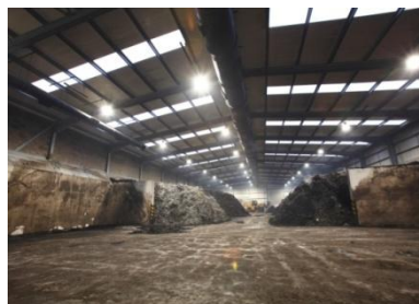
In-Vessel Composting (IVC) facility at Chichester Street in Rochdale
