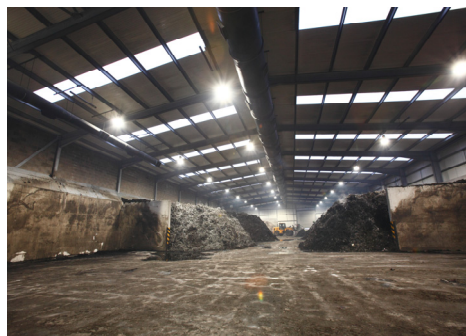
In-Vessel Composting (IVC) facility at Chichester Street in Rochdale
