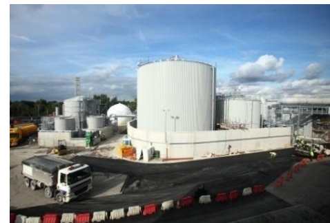
Mechanical and Biological Treatment and Anaerobic Digestion facility at Reliance Street in Manchester - the first one to be completed.
